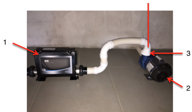
1. Elbox 2. Pump 3. Snabbkoppling
